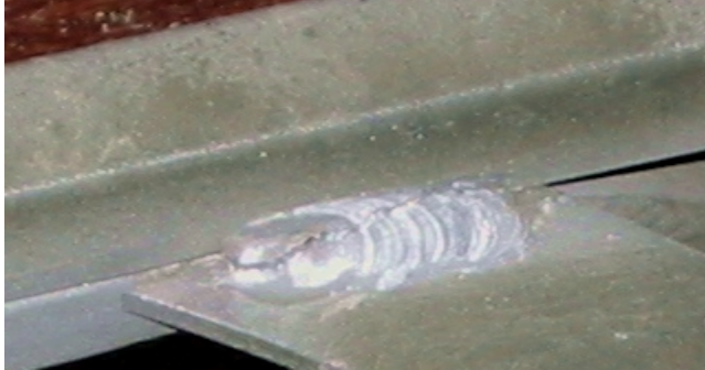
Figure 14. Picture of a Crater Crack (by Paul Cameron, Public Domain)
