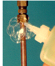
Figure 33. Leak Testing (by Paul Phelps, CC BY-SA 4.0)
