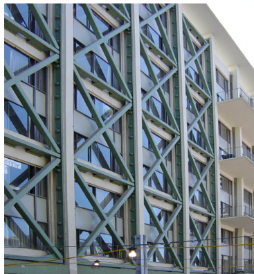
Figure 11 Shear Trusses (by Leonard G, CC SA 1.0)
