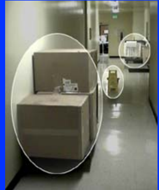
Obstructed exit route
